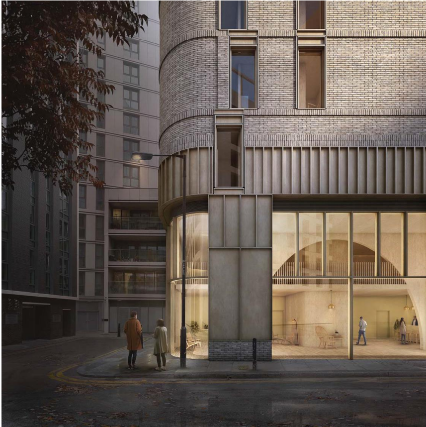
Figure 3: CGI of glazed ground and 1 st (mezzanine) floor incorporating rusticated nickel cladding finish to base with soldier course brick detail set above
